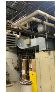
EXISTING HEAT PUMP SUPPLY VENTILATION
