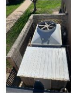
EXISTING COOLING TOWER & PUMP SHED
