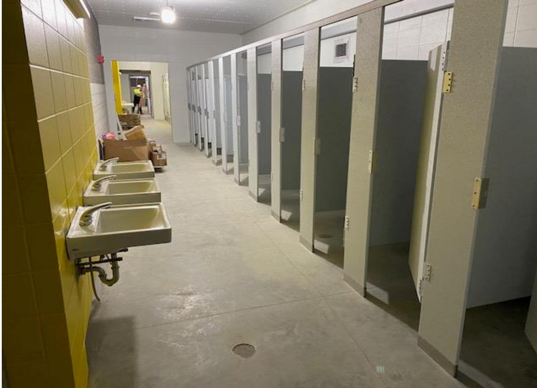
Restroom partitions on east and west complete
