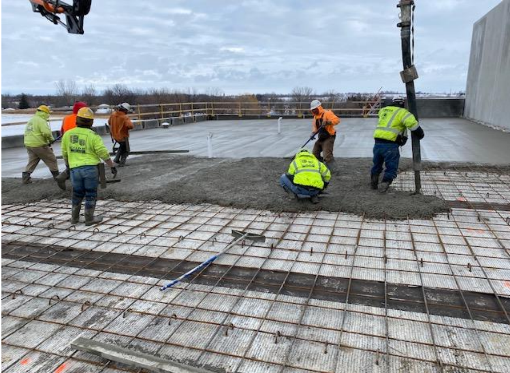
Concrete pouring over locker rooms
