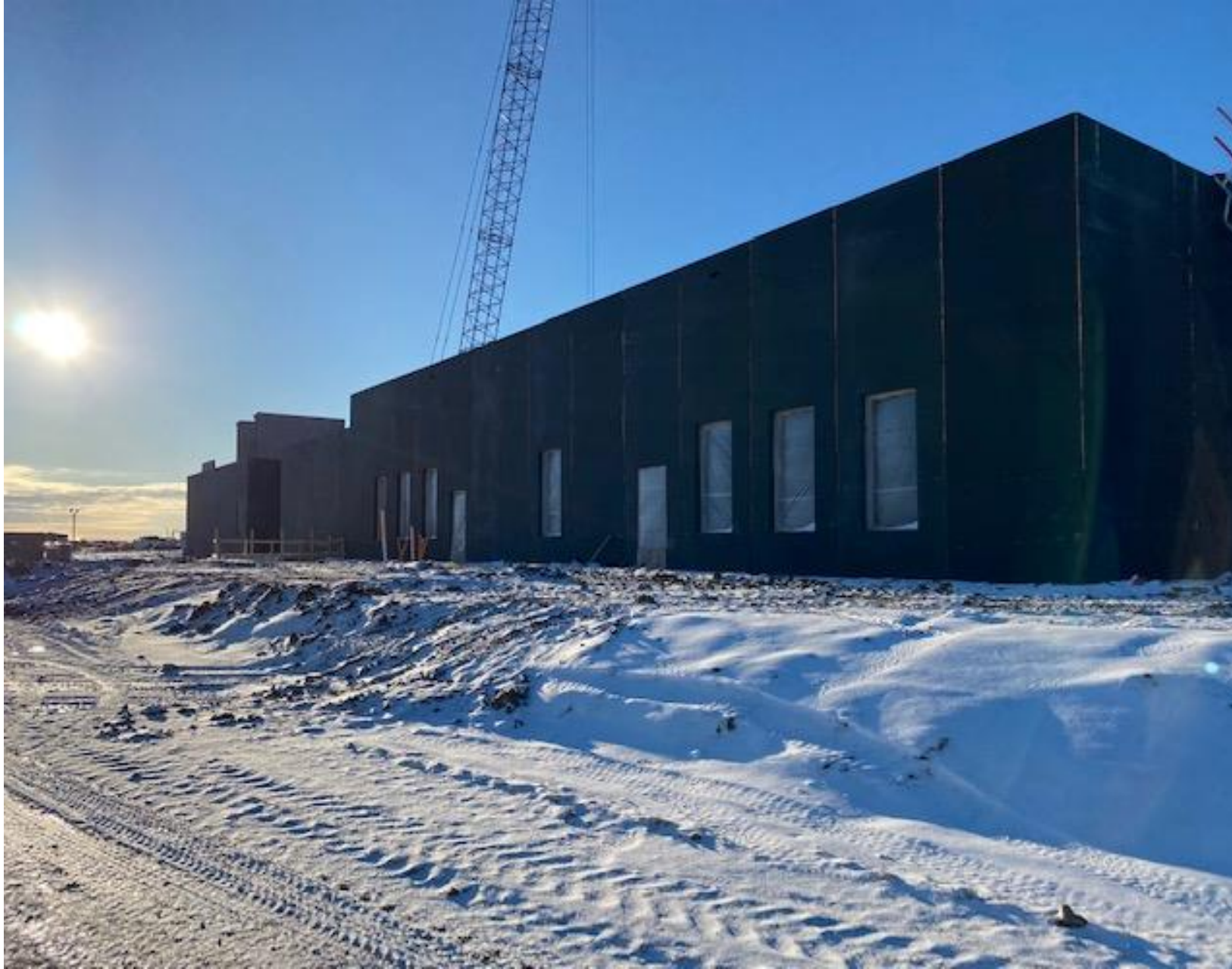
North wall of Multipurpose/Wrestling
