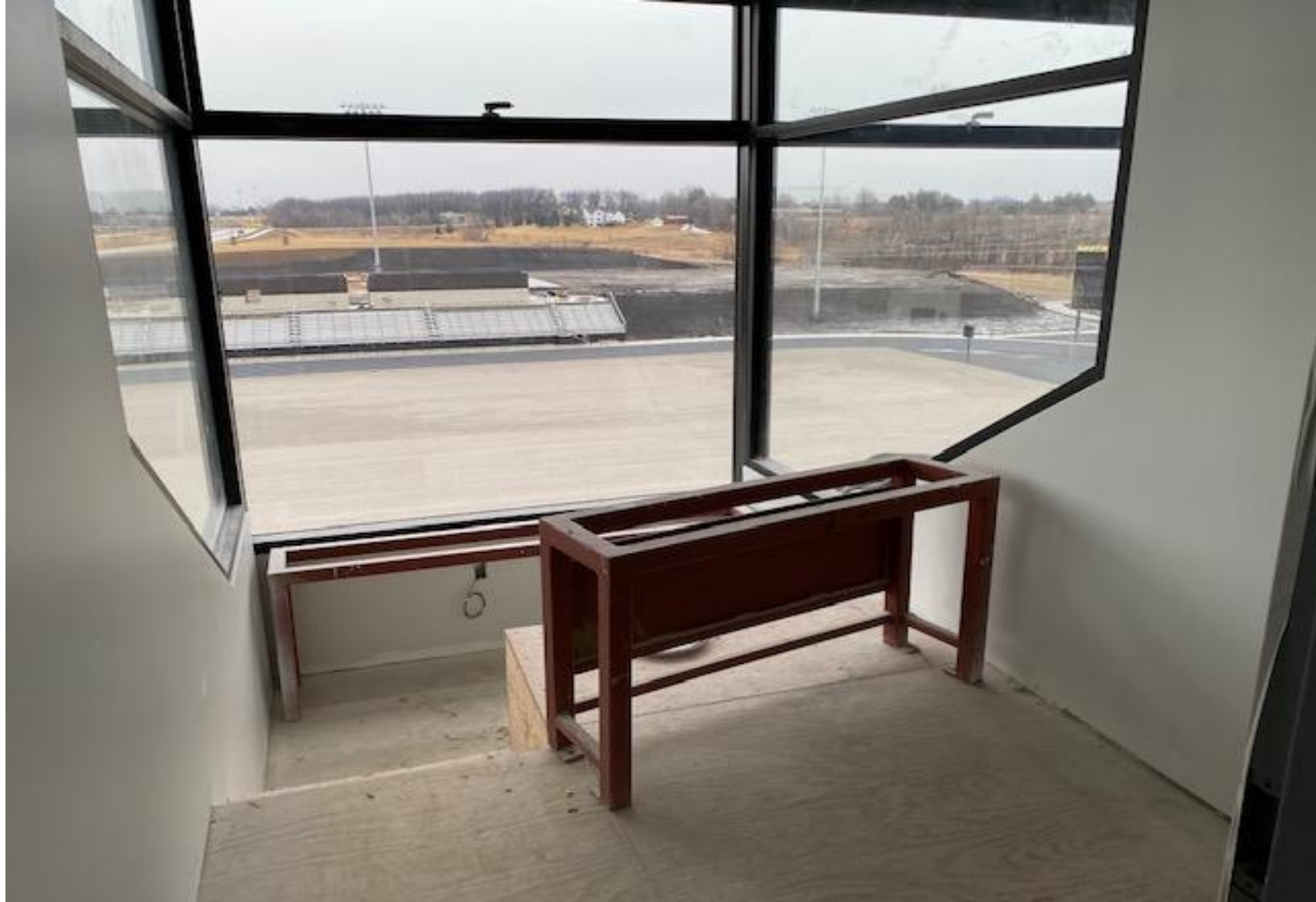
Interior finishes progress in press box
