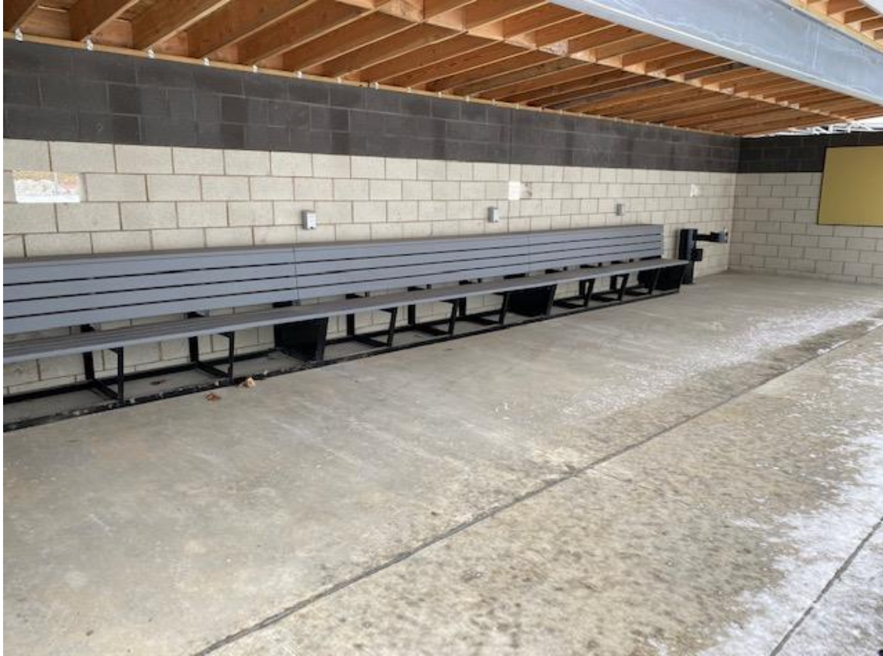
Softball dugout progress
