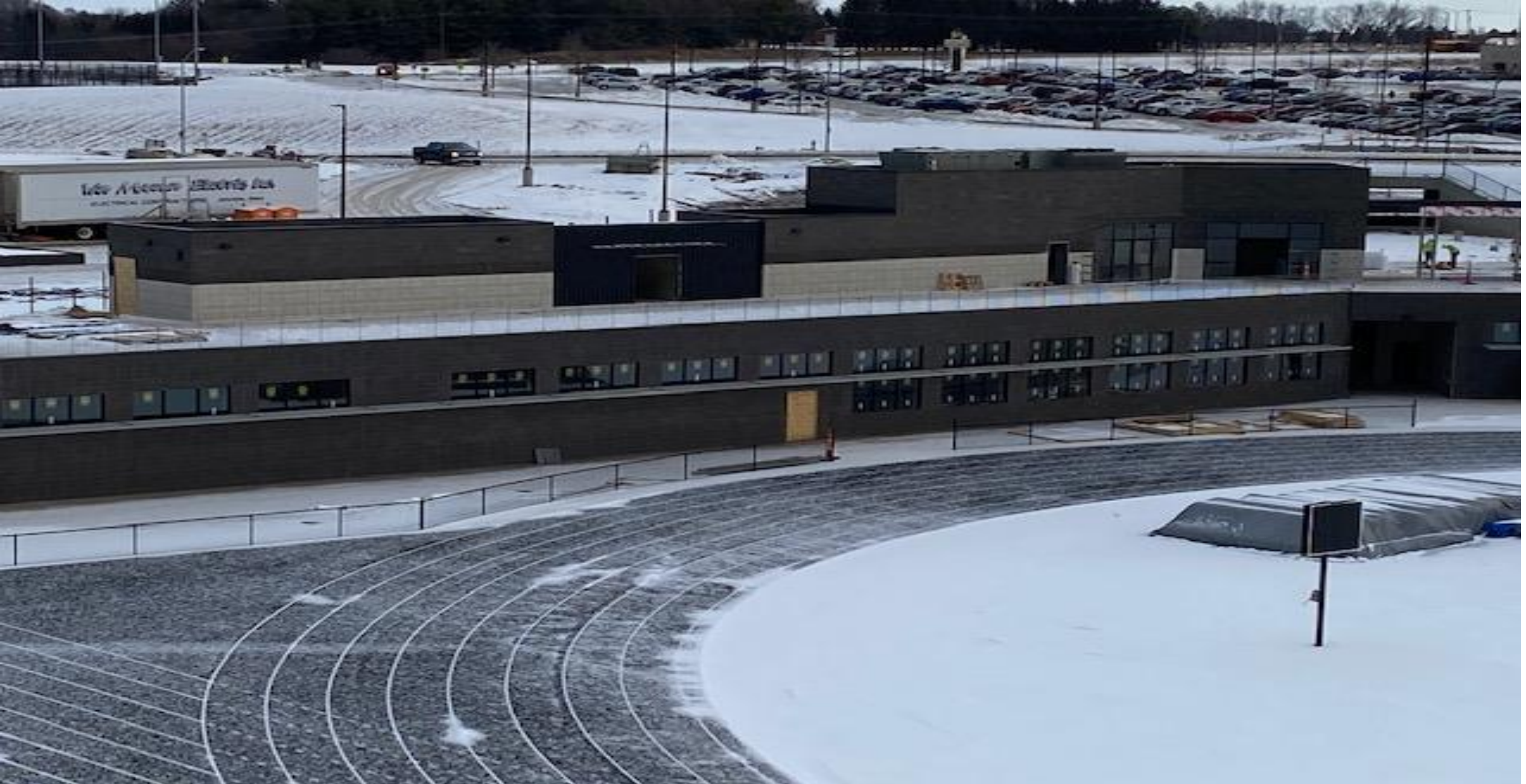
North lower-level windows installed
