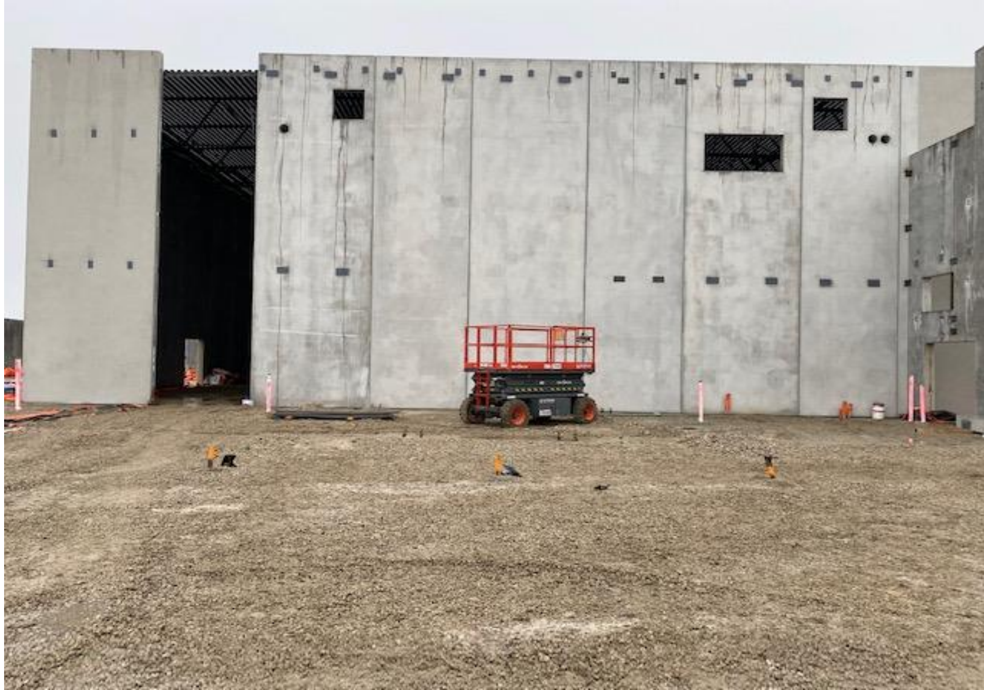
East wall of Gym
