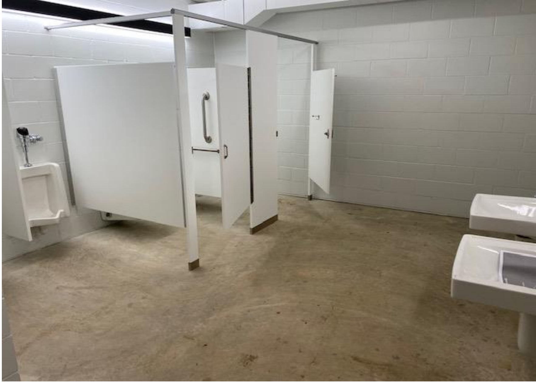
Restrooms nearly complete
