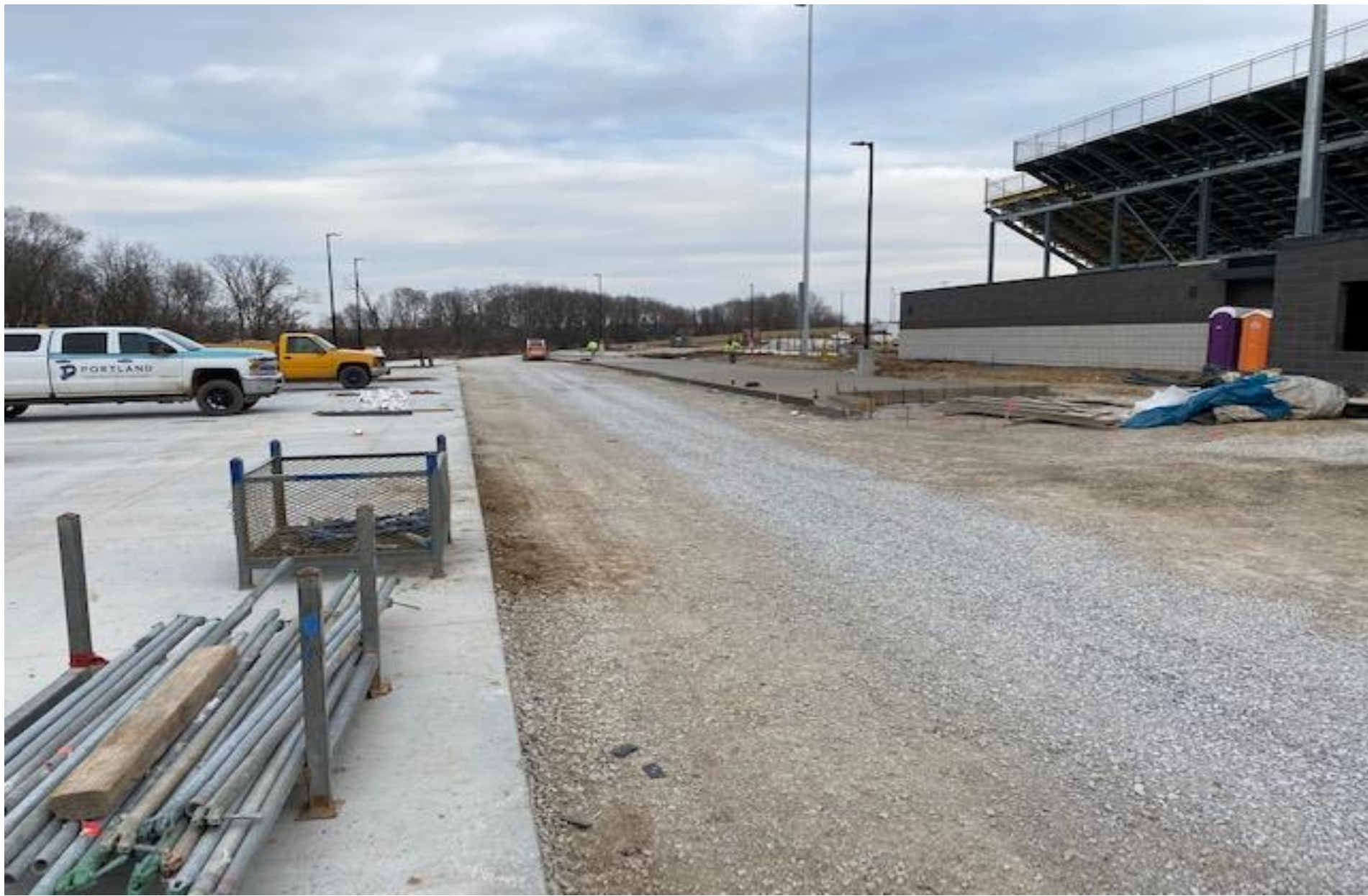
Paving continues west of bleachers.
