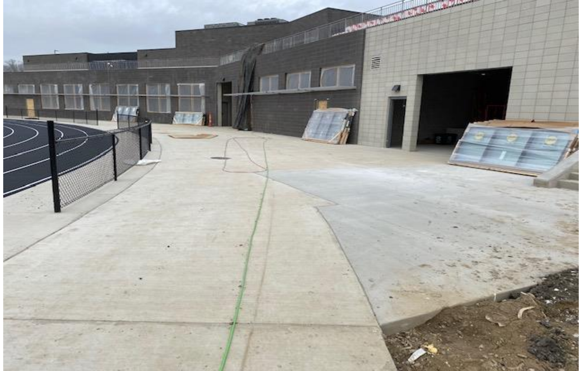
Windows ready for installation.
