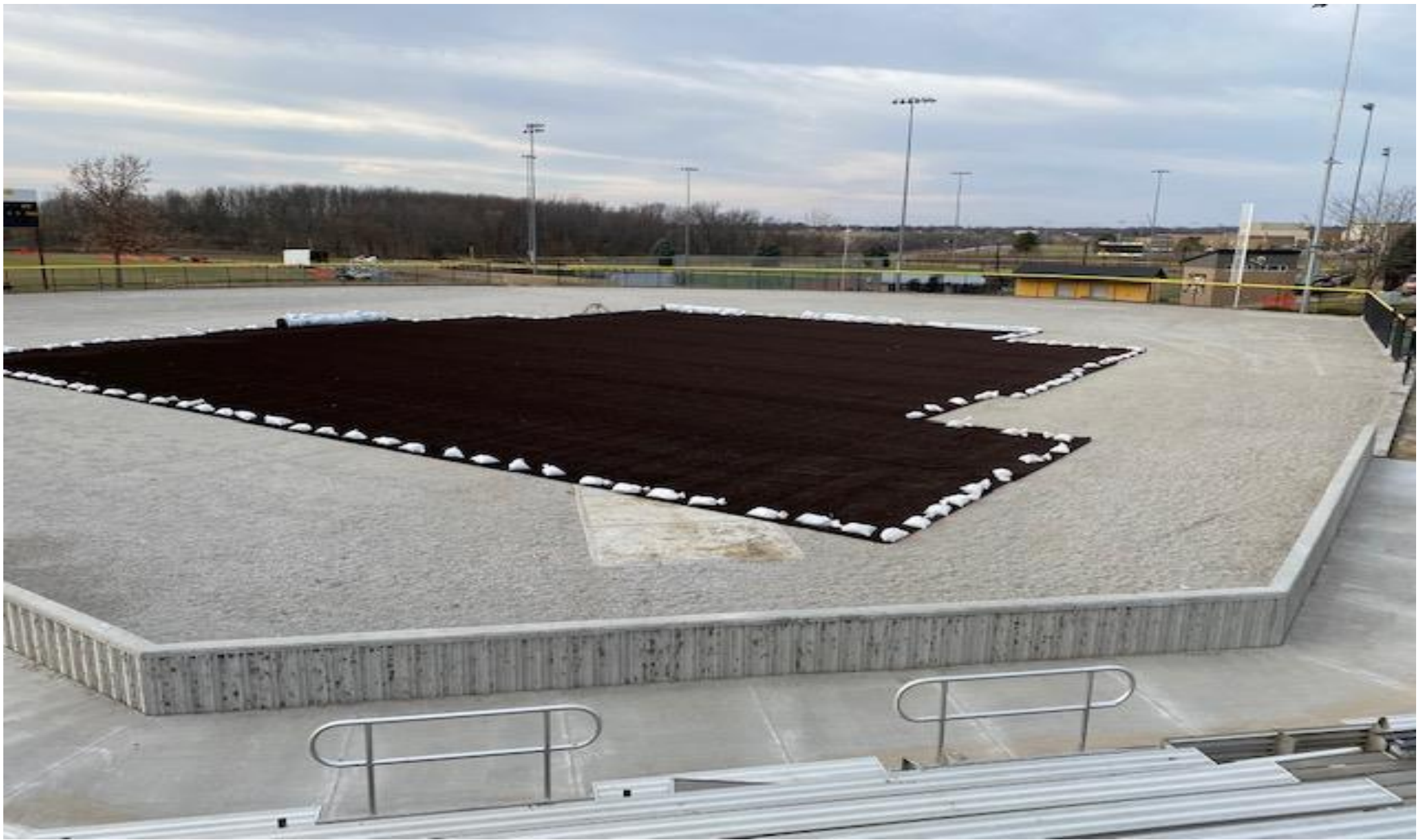
Partial install of softball turf
