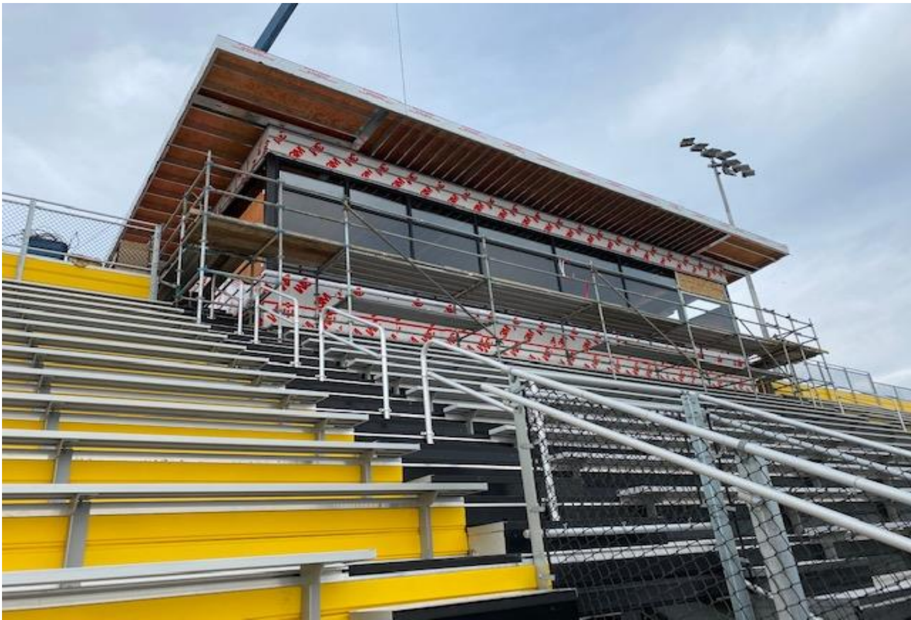
Press box progress.
