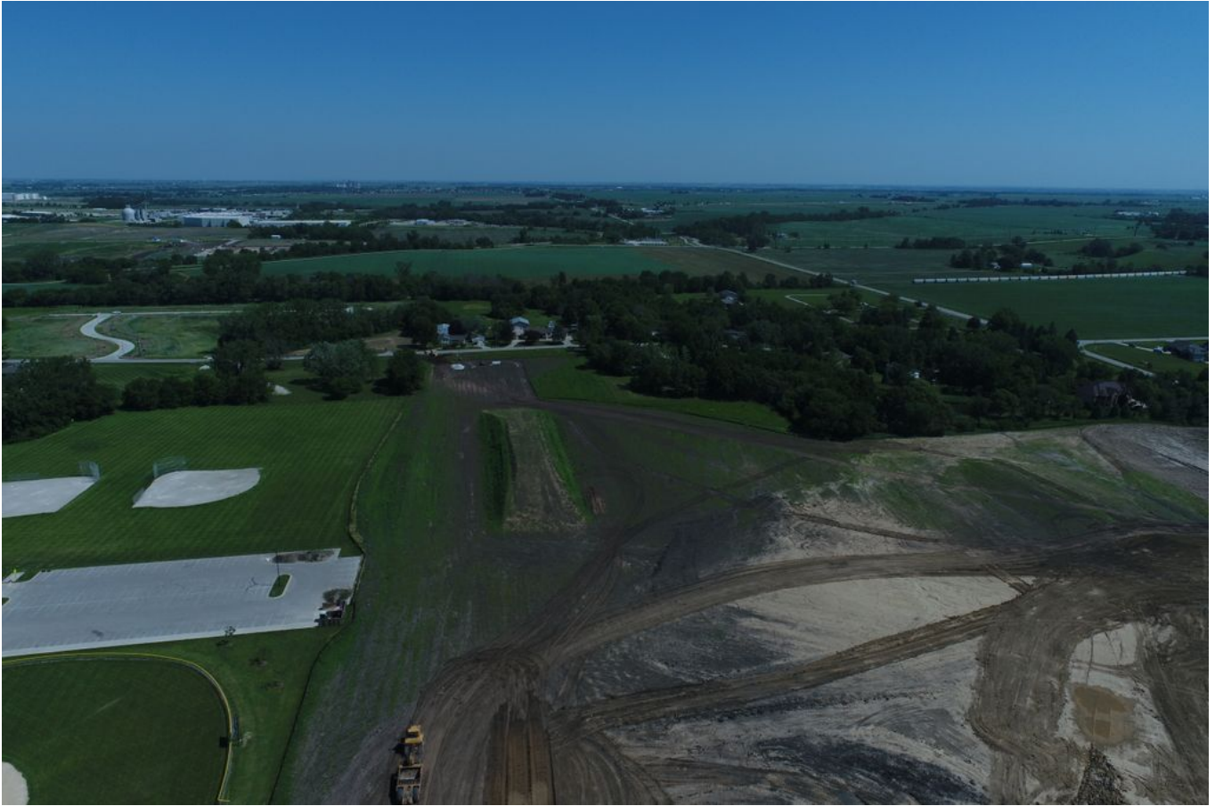
Middle of west side, looking north
