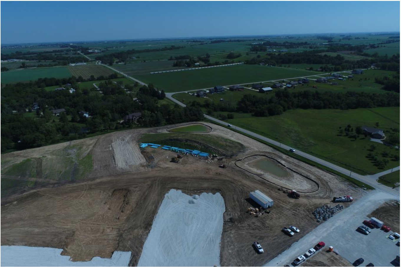
Above building pad, looking to NE corner of site
