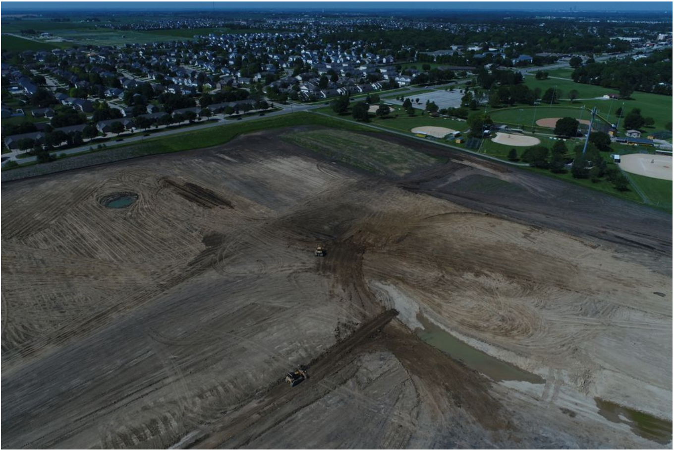
Above building pad, looking SW
