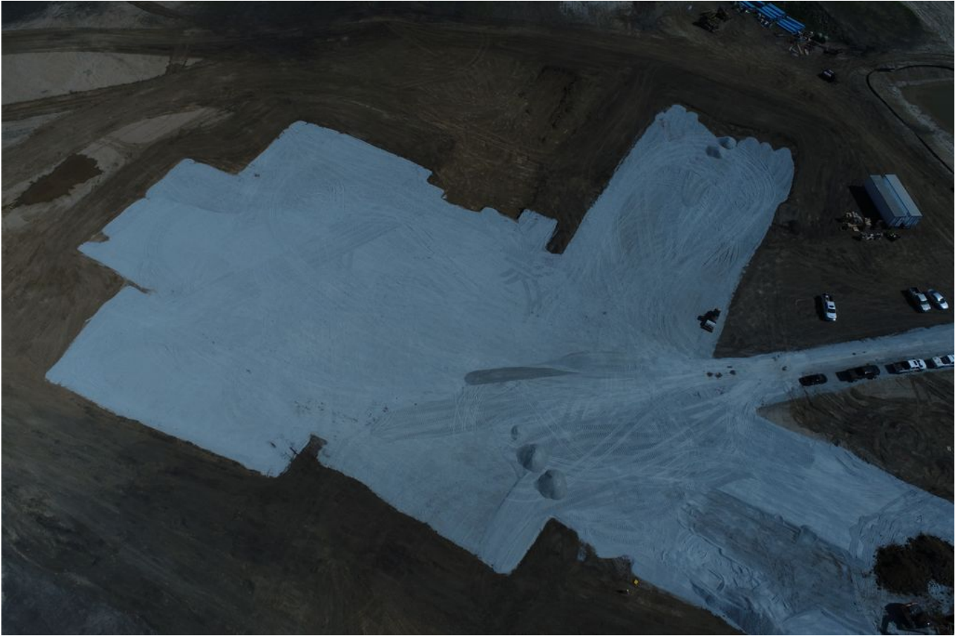
Building pad, from slightly south
