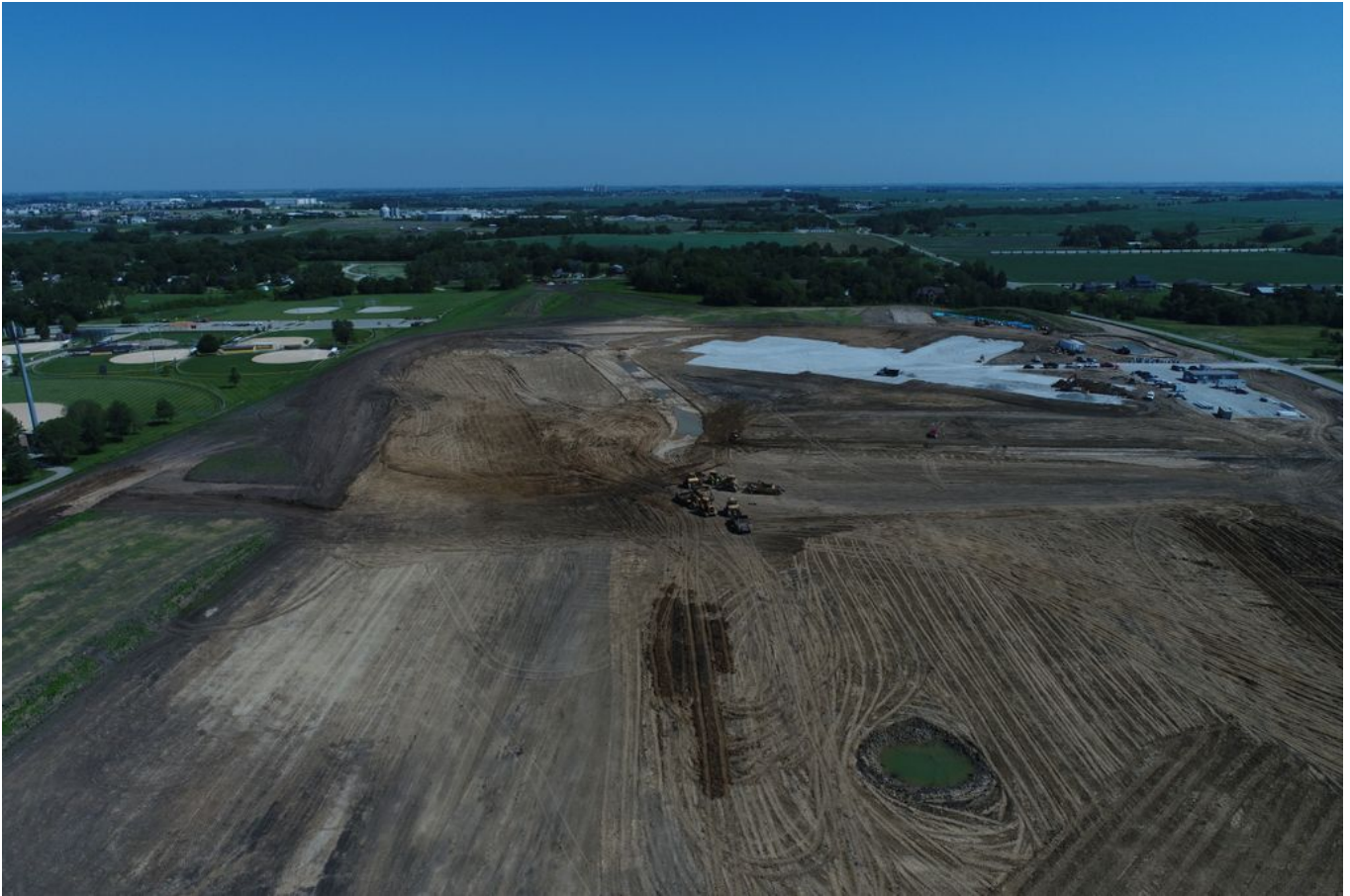
Middle of south end, looking north
