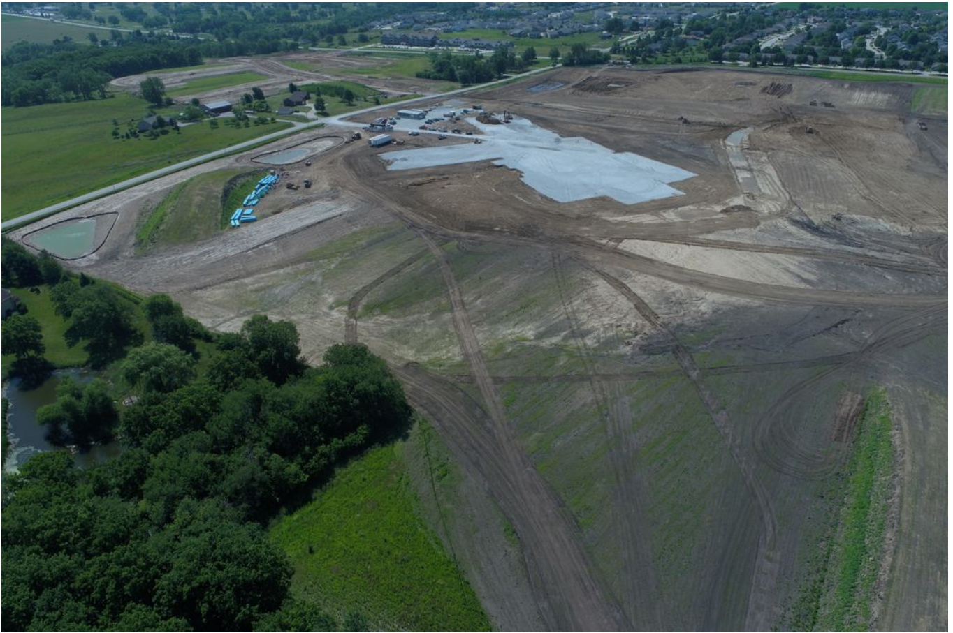
NW corner of site, looking toward building pad
