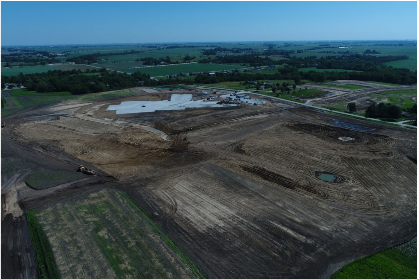
SW corner, looking toward building pad
