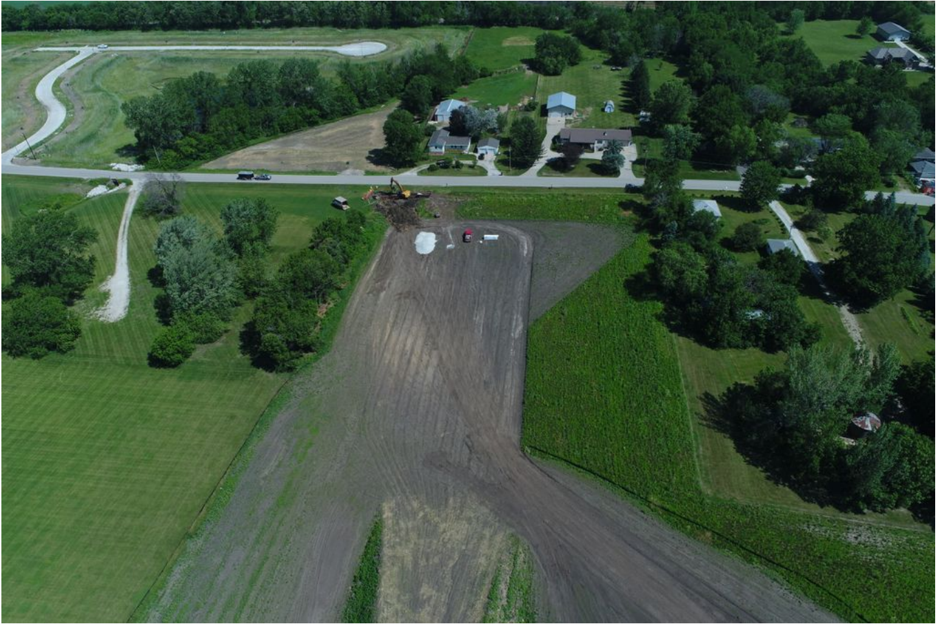
NW corner of site; septic tank work
