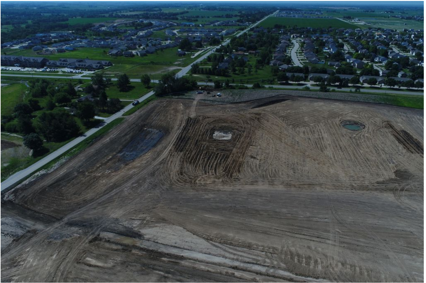
Above building pad, looking south
