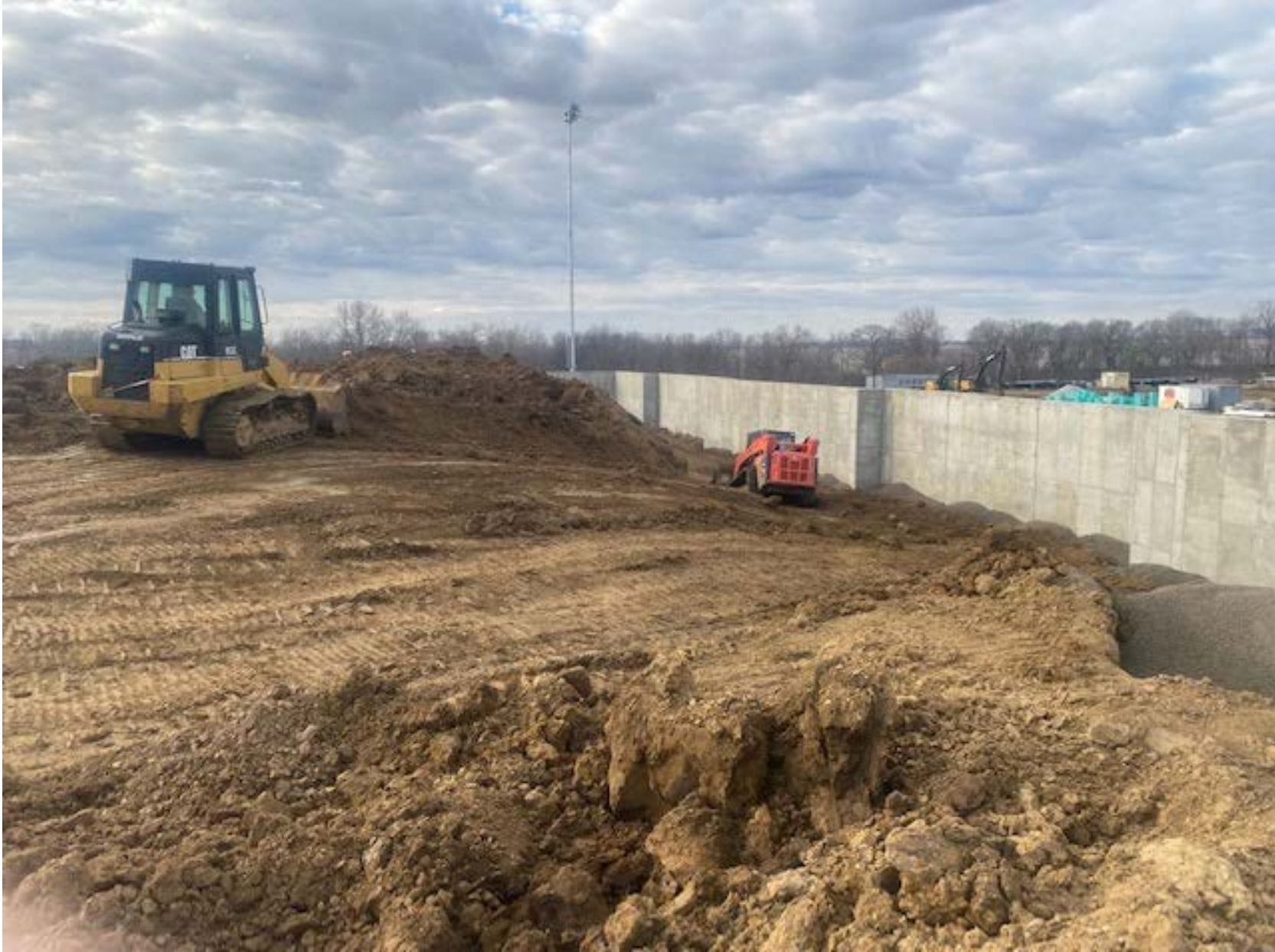
East side backfill behind retaining wall
